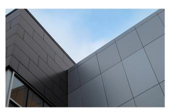
**Joint seals on exterior wall cladding.** Weather resistant and self-adhesive EPDM strips are installed at the edge of facade panels to absorb minor tolerances in the structure. They also seal off the structure from ingress of dirt and water, guiding the flow of rain to the outside of the building envelope.
